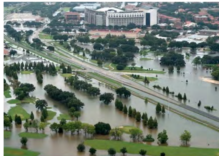
CAMPUS FLOODING AUGUST 2016
