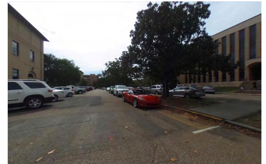
EXISTING WEST QUAD PARKING LOT
