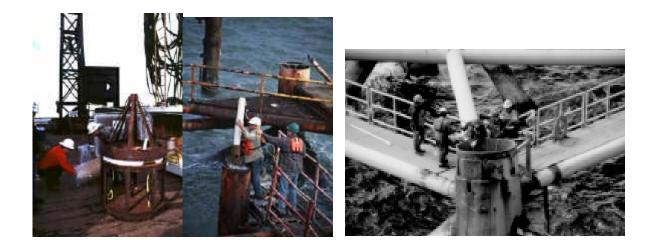
Figure C.6. Explosives Technicians Prepare and Load Charges into Conductors and Legs (National Marine Fisheries Service – Galveston, 2004).
