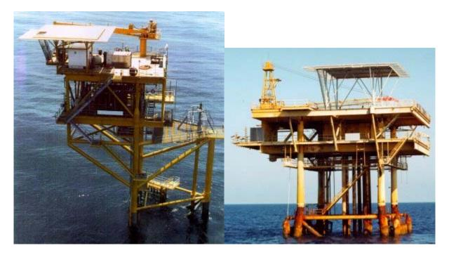
Figure E.2. Well Protector Structures in the Gulf of Mexico (Twachtman Snyder and Byrd, Inc., 2006).
