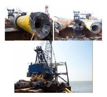
Figure C.7. Severed Piles and Conductors Loaded Onto Derrick Barge (DEMEX, 2004).
