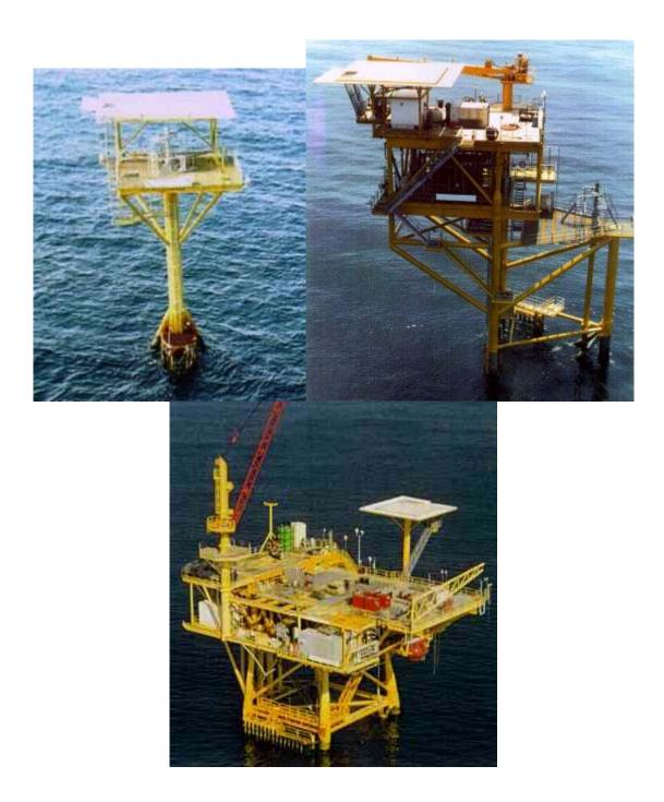
Figure A.2. Caisson, Well Protector, and Fixed Platform Structures (Twachtman Snyder & Byrd, Inc., 2006).
