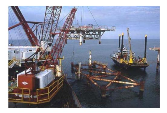
Figure C.4. Derrick Barge Arrives On-Site and Removes the Deck Module (National Marine Fisheries Service – Galveston, 2004).
