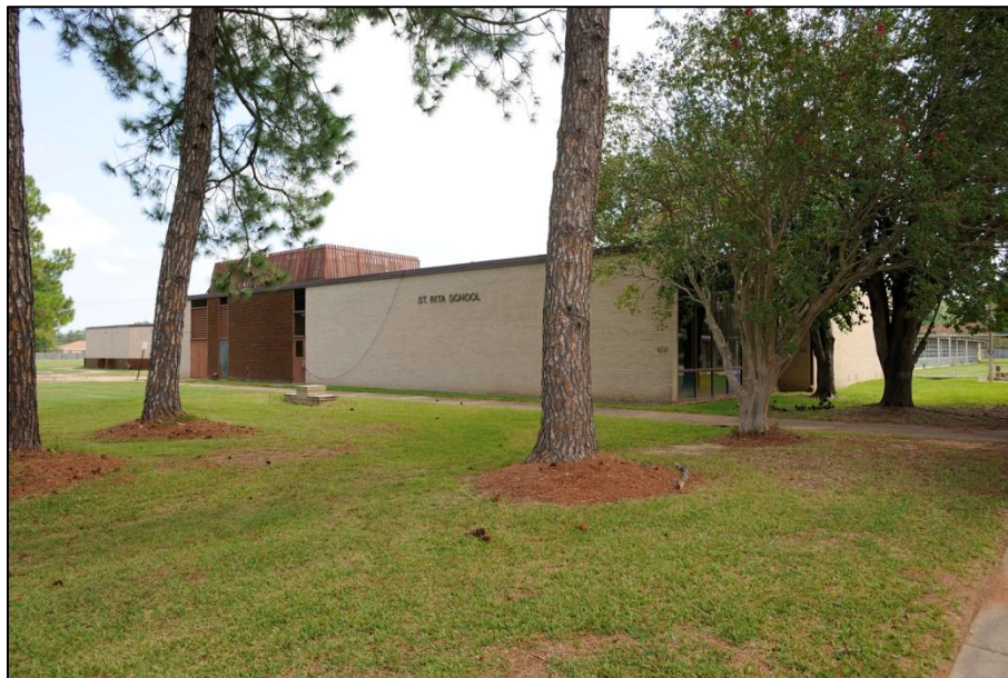
FIGURE B2: St Rita’s Elementary School, 2386 Vandenburg Dr, England Airpark
