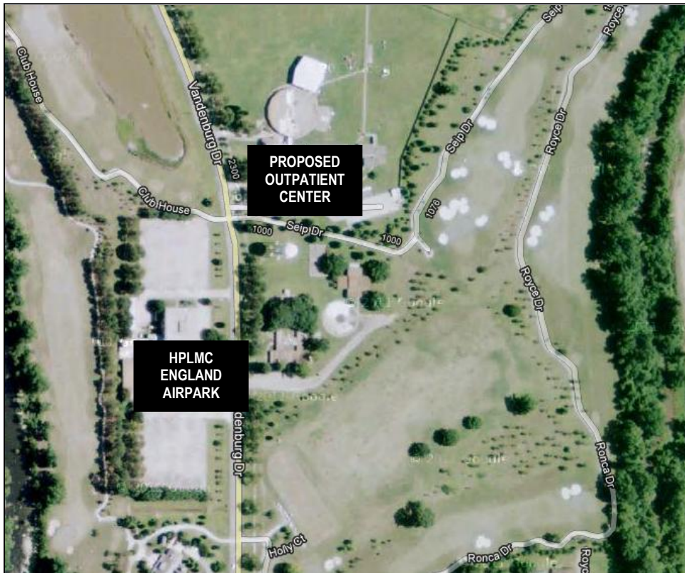
FIGURE B4: Aerial view of the HPLMC Airpark Facility
